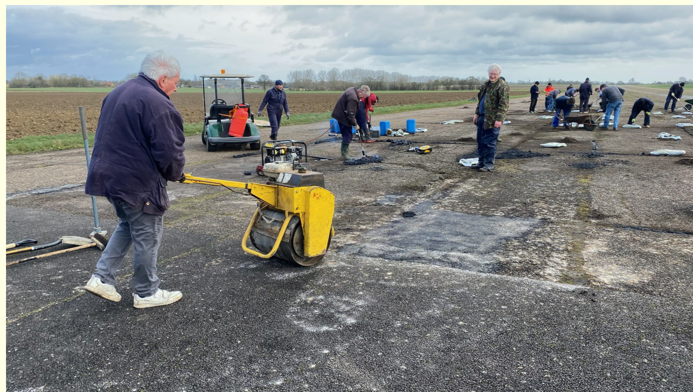
RGC runway repair crew
